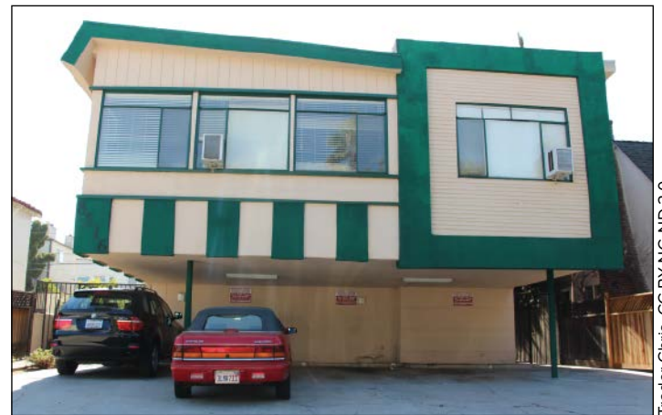
A “dingbat” apartment in Los Angeles, characterized by an overhang sheltering street-front parking. Popular in the 1950s and 1960s, these types of structures are particularly vulnerable to collapse during earthquakes.
