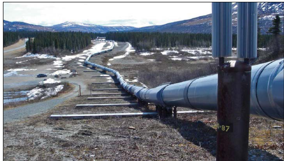
Trans-Alaska oil pipeline crossing the Denali Fault.
