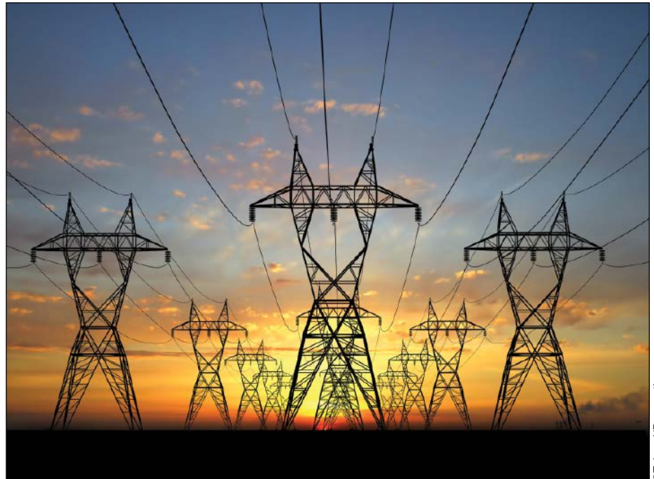
Fig. 1. Electric power lines at sunrise.
