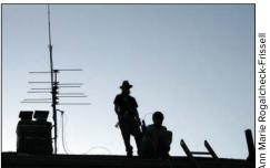
Joseph Przebieglec (left; ham radio call sign KC2NSS) and Nathaniel Frissell (right; call sign W2NAF) install a simple G5RV-type wire antenna on the roof of a house. Simple antennas such as these allow amateur radio operators around the world to transmit on high frequencies and contribute to data collected by the Reverse Beacon Network and other real-time amateur radio reporting networks.
