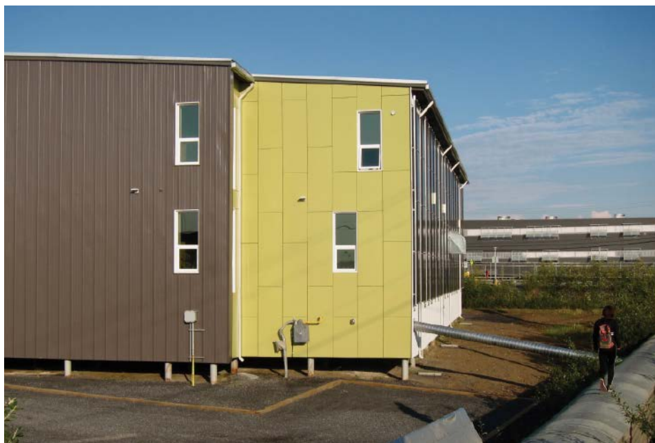
Many buildings in Inuvik and across the Arctic use traditional steel pilings as a foundation. Each pillar is filled with a slurry of gravel, sand, and mud that freezes in cold weather and then helps keep the permafrost in which it is buried frozen as the region warms again in the spring and summer. Credit: Laura Poppick
