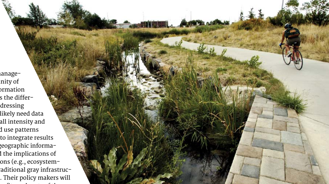
A flood mitigation method in Boulder, Colo., uses a basinlike shape bounded by rock walls that should contain rising water on the Goose Creek pathway. Credit: Marty Caivano/Digital First Media/Boulder Daily Camera via Getty Images
