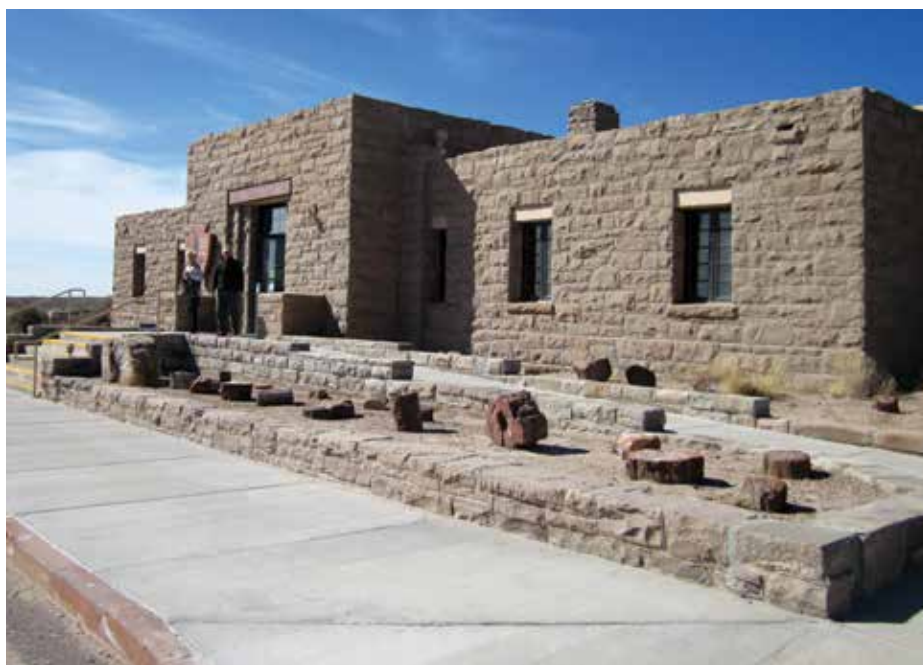
The access ramp leading up to the front entrance to the Rainbow Forest Museum at the Petrified Forest National Park was made with natural sandstone to match the original 1931 building. Credit: NPS/Hallie Larsen
