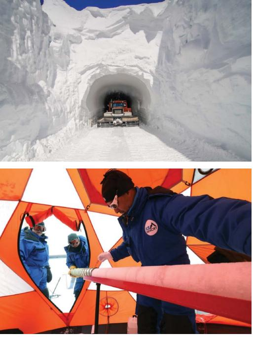
(top) Constructing giant trenches at Dome Concordia in Antarctica. Digging these trenches was the first step in trialing how to store ice cores in underground caves. Credit: Armand Patoir, French Polar Institute IPEV (bottom) Ice Memory project scientists extract ice cores at Illimani glacier in Bolivia in 2017 Credit: Sarah Del Ben, Foundation Grenoble Alpes University
