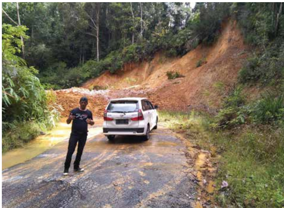
Heavy rainfalls in June 2020 triggered a landslide that covered roughly 50 meters of roadway in Geumpang, Aceh, Indonesia. Credit: Andrean Simanjuntak
