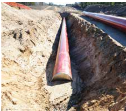
A new pipeline is installed in 2009 through the Bemidji oil spill site in Minnesota. Credit: Andrew Berg
