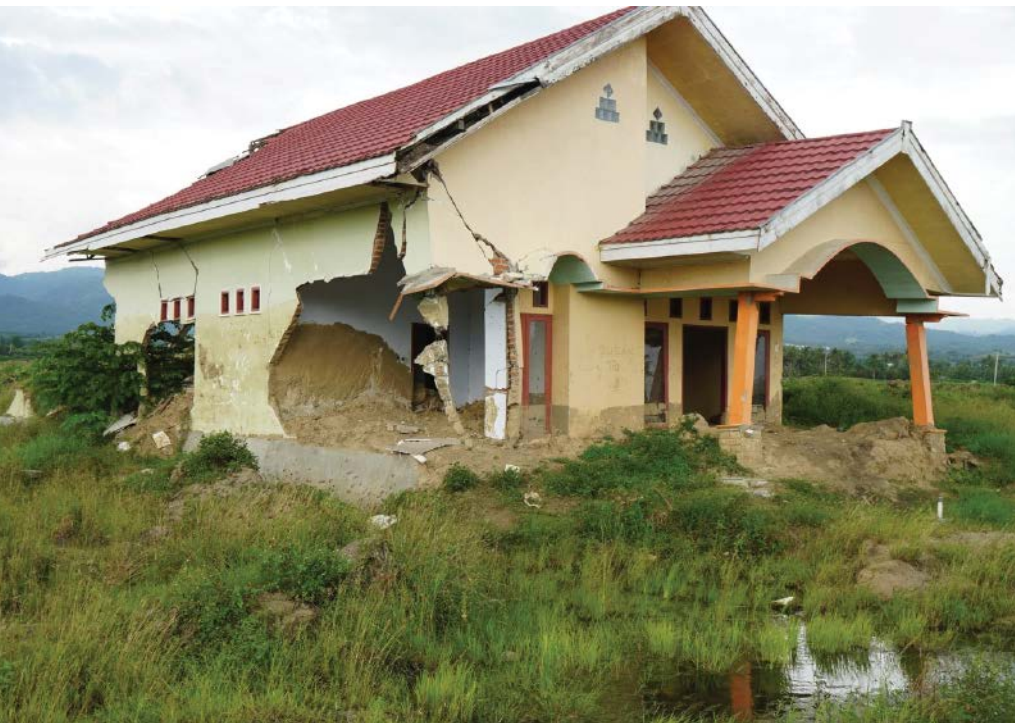
A house in Palu, Indonesia, stands on a liquefied foundation following the devastating 2018 Sulawesi earthquake. Seismologists are investigating whether crowdsourced, firsthand accounts of earthquakes could help determine the appropriate response to quakes like this. Credit: Walter Mooney, USGS
