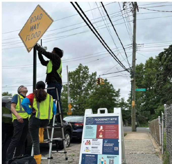
Members of the FloodNet team install a sensor designed to provide real-time flood information to community members, researchers, and agencies in New York City. Credit: Veronique Ignace
