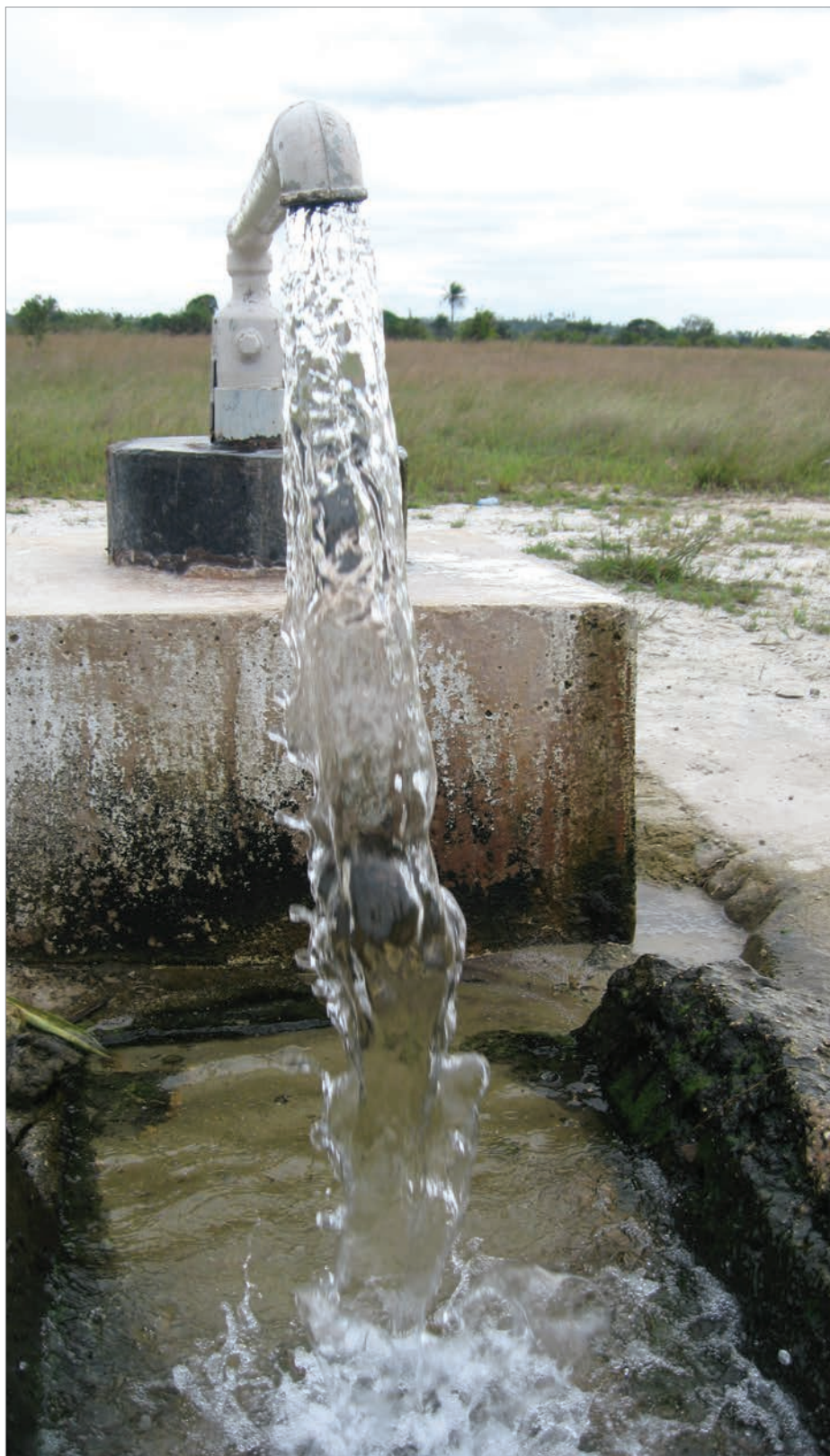
Water flows from a well drilled roughly 600 meters underground into the Kimbiji Aquifer in Tanzania. Credit: Ruden AS
