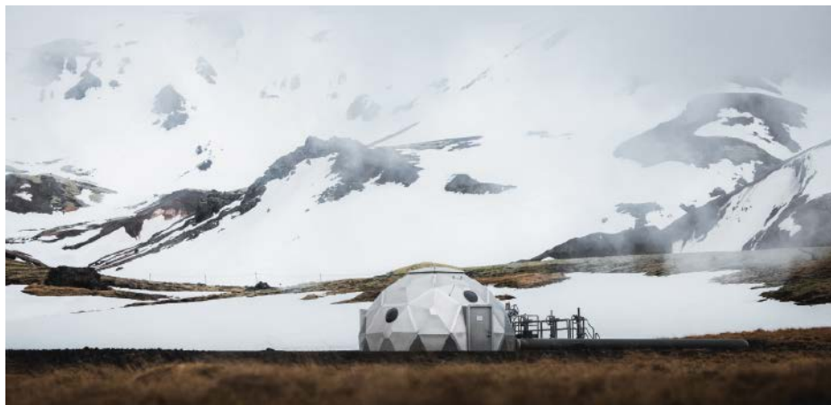
At sites like this one, the Icelandic company Carbfix injects carbon dioxide dissolved in water into underground geologic reservoirs, where it reacts with rock to form carbonate minerals. Credit: Siljaye/Wikimedia Commons, CC BY-SA 4.0 ( bit.ly/ccby4-0 )
